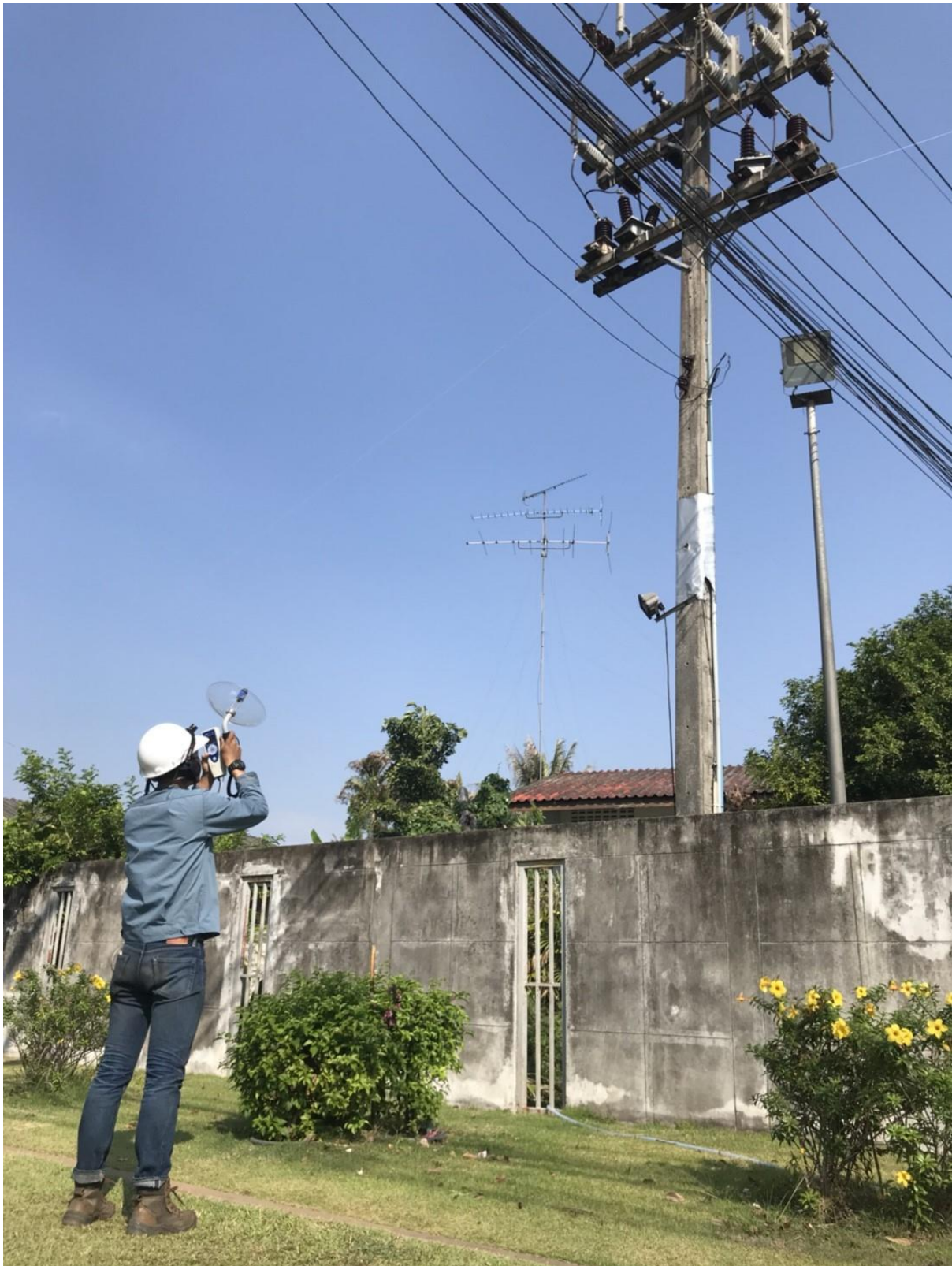
PD TEST BY ULTRADISH MODE AT 22 kV DISTRIBUTION POLE METERING
