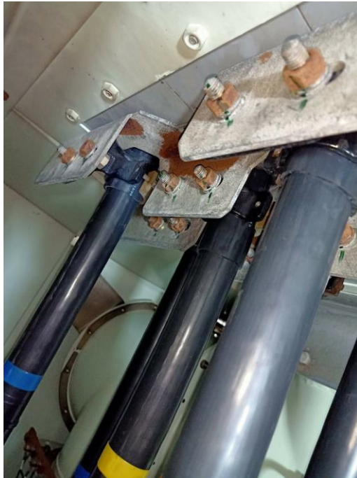
PARTIAL DISCHARGE DETECTED BY VISUALLY INSPECT
