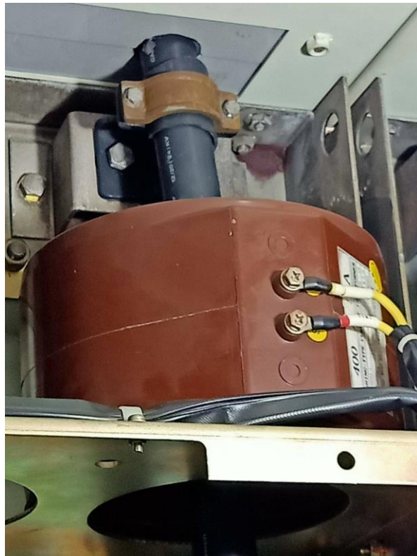
PARTIAL DISCHARGE DETECTED BY VISUALLY INSPECT
