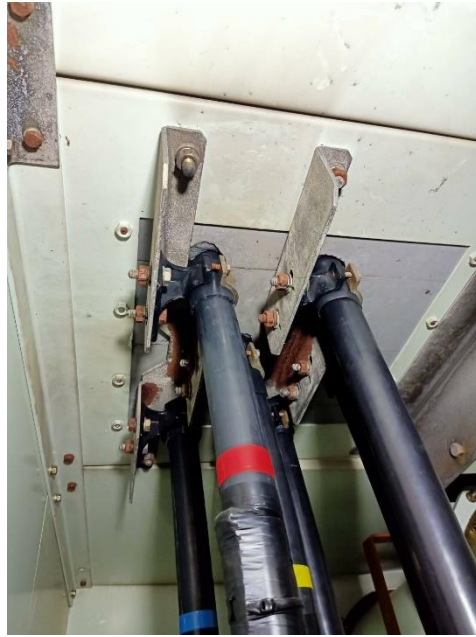
PARTIAL DISCHARGE DETECTED BY VISUALLY INSPECT
