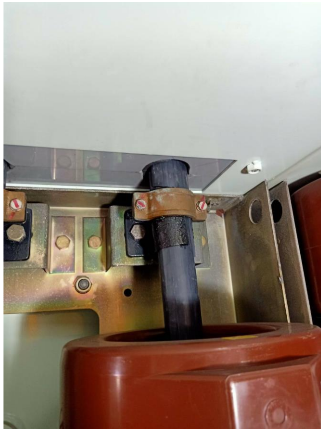
PARTIAL DISCHARGE DETECTED BY VISUALLY INSPECT
