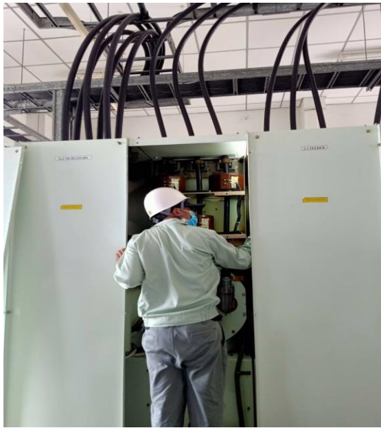
PARTIAL DISCHARGE DETECTED BY VISUALLY INSPECT
