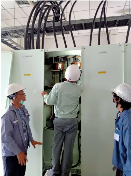
PARTIAL DISCHARGE DETECTED BY VISUALLY INSPECT
