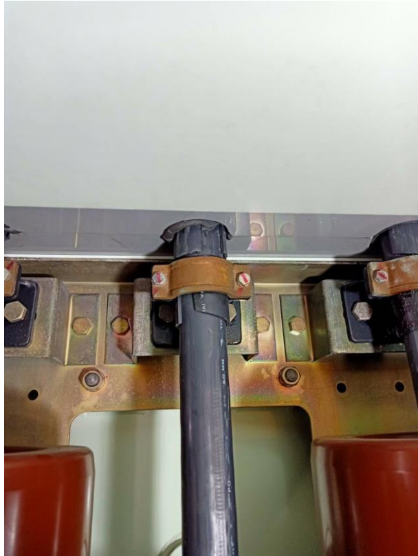
PARTIAL DISCHARGE DETECTED BY VISUALLY INSPECT
