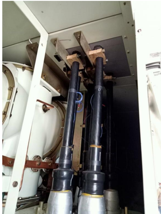
PARTIAL DISCHARGE DETECTED BY VISUALLY INSPECT
