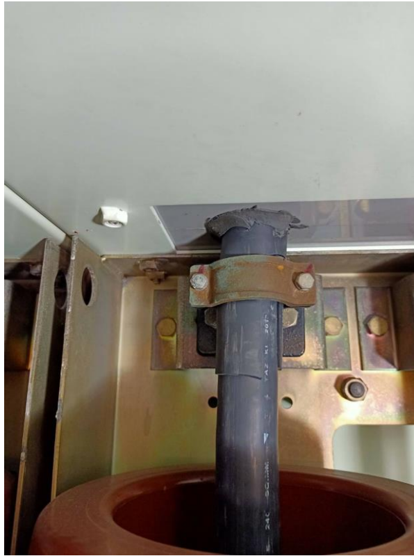
PARTIAL DISCHARGE DETECTED BY VISUALLY INSPECT
