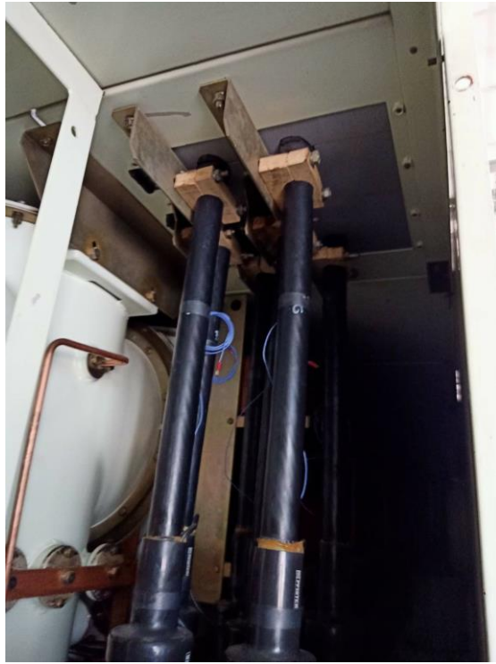
PARTIAL DISCHARGE DETECTED BY VISUALLY INSPECT
