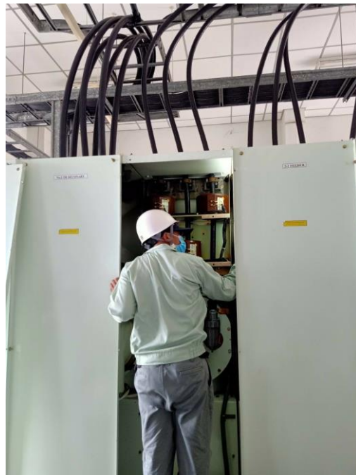
PARTIAL DISCHARGE DETECTED BY VISUALLY INSPECT
