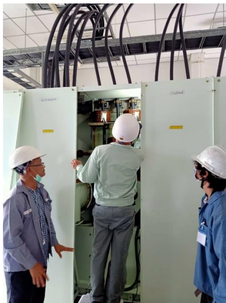
PARTIAL DISCHARGE DETECTED BY VISUALLY INSPECT
