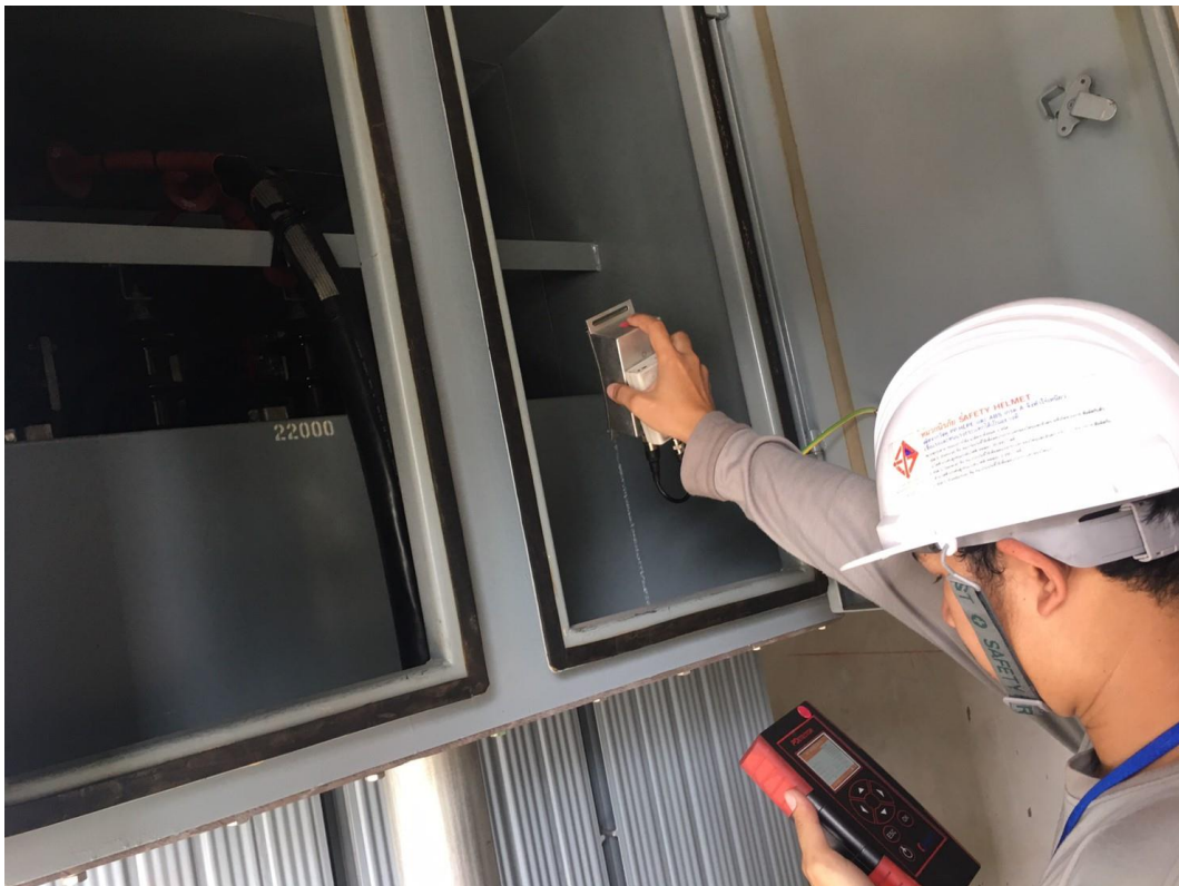
PHOTO 6 : PARTIAL DISCHARGE INSPECTION BY UHF MODE
