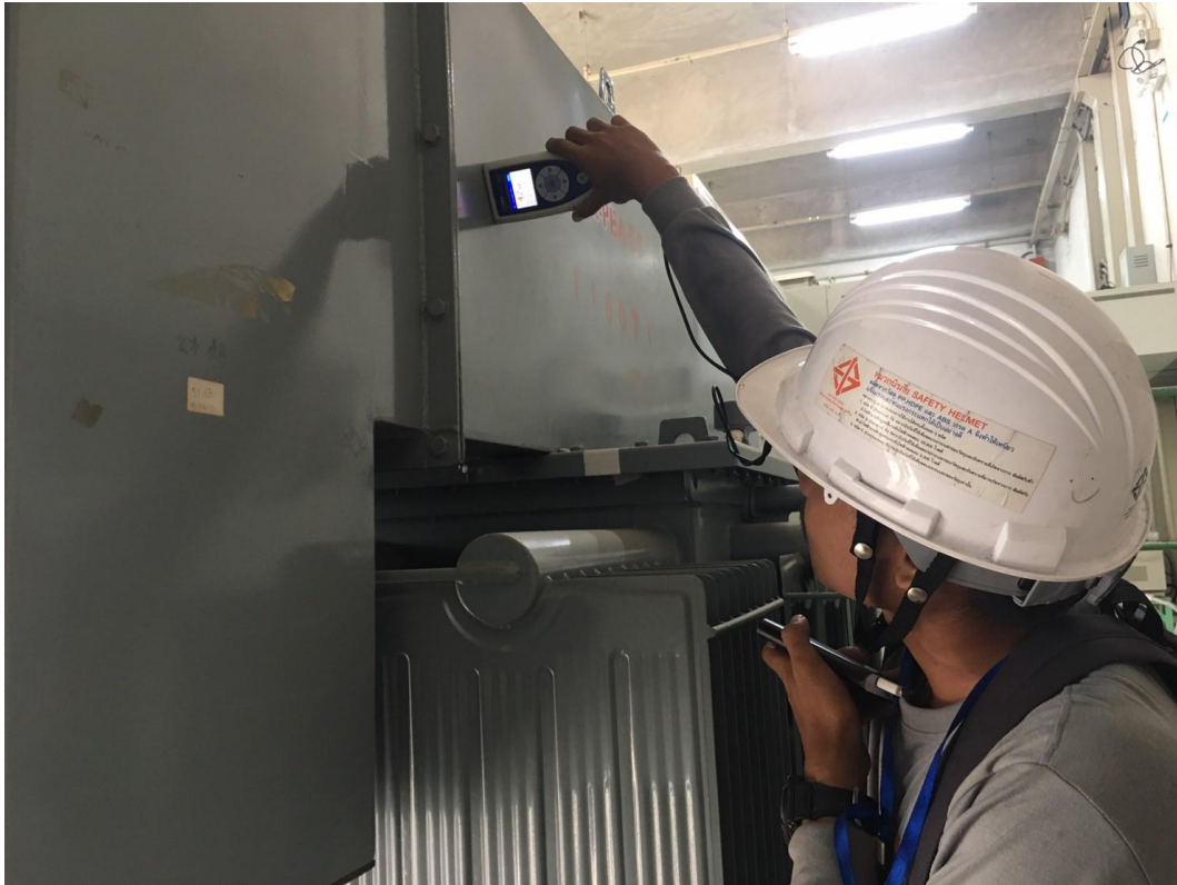
PHOTO 3 : PARTIAL DISCHARGE INSPECTION BY TEV MODE
