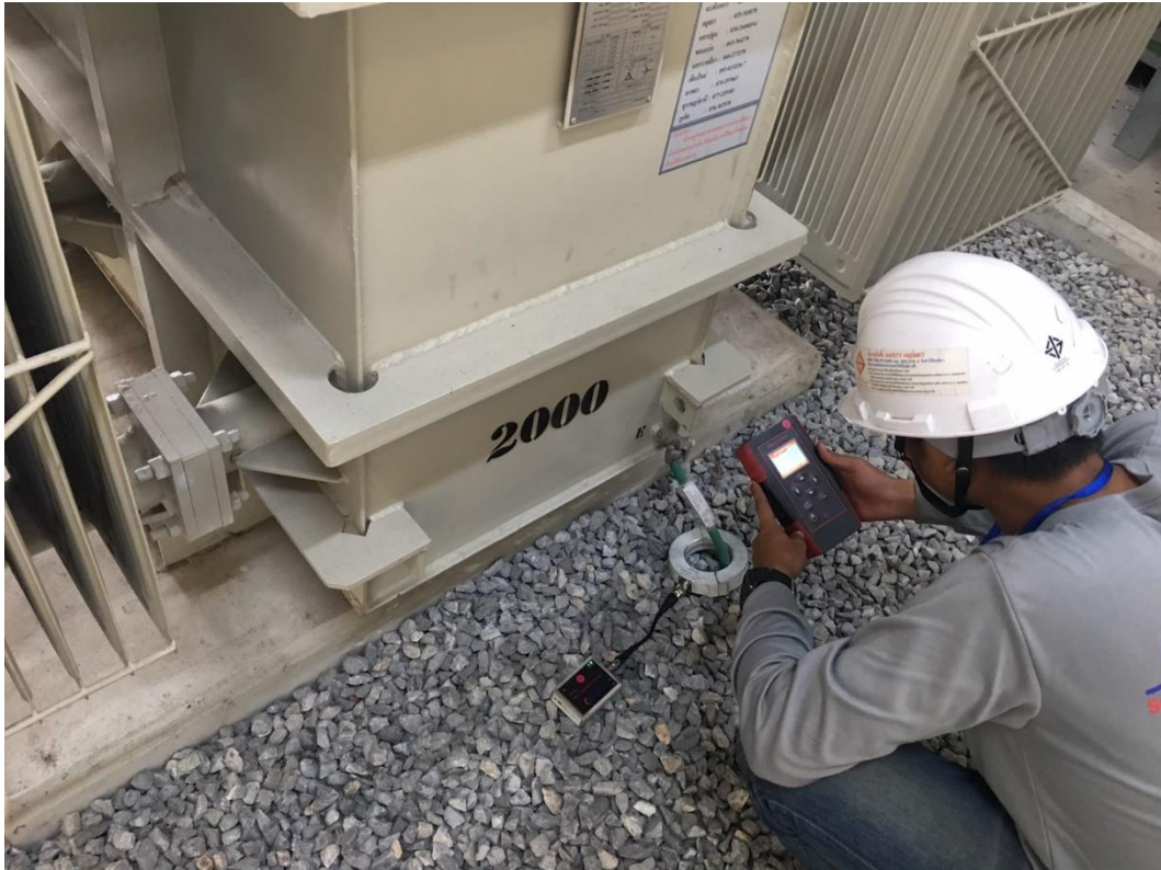
PHOTO 7 : PARTIAL DISCHARGE INSPECTION BY HFCT MODE
