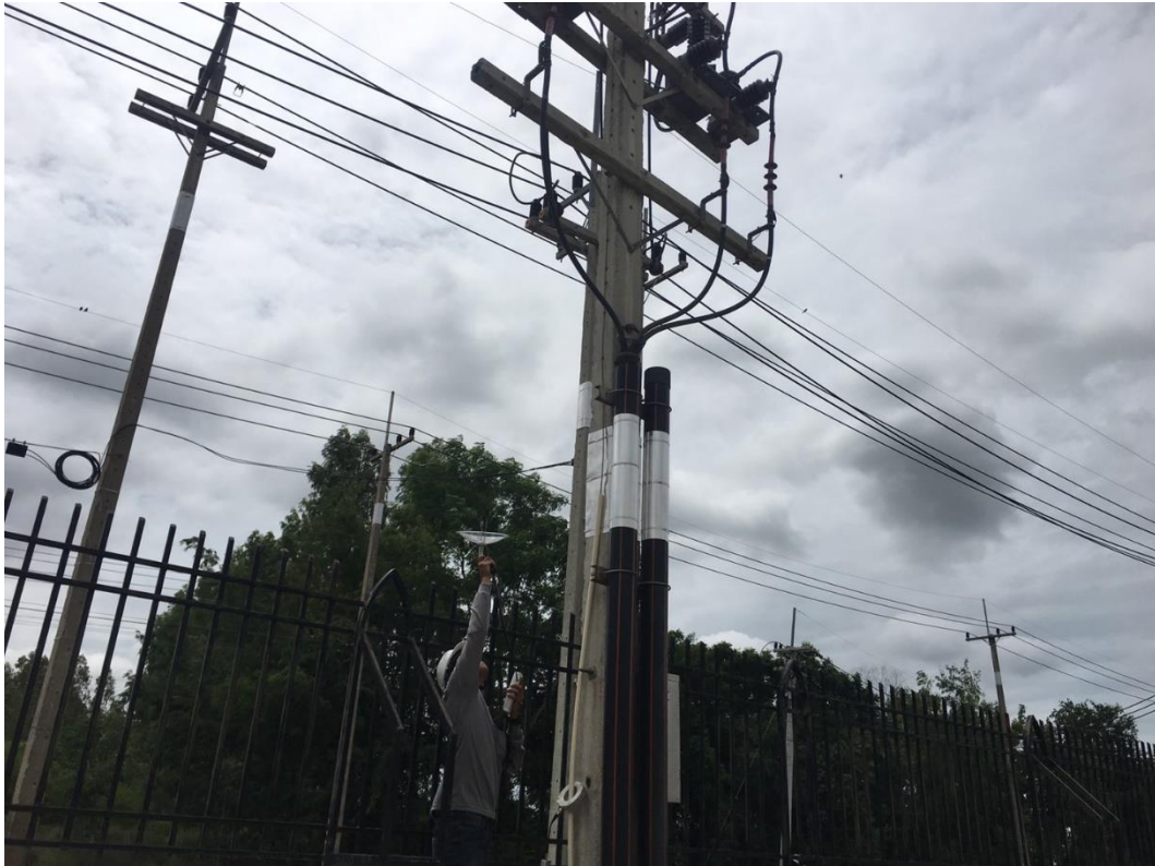
PHOTO 1 : PARTIAL DISCHARGE INSPECTION BY ULTRADISH MODE
