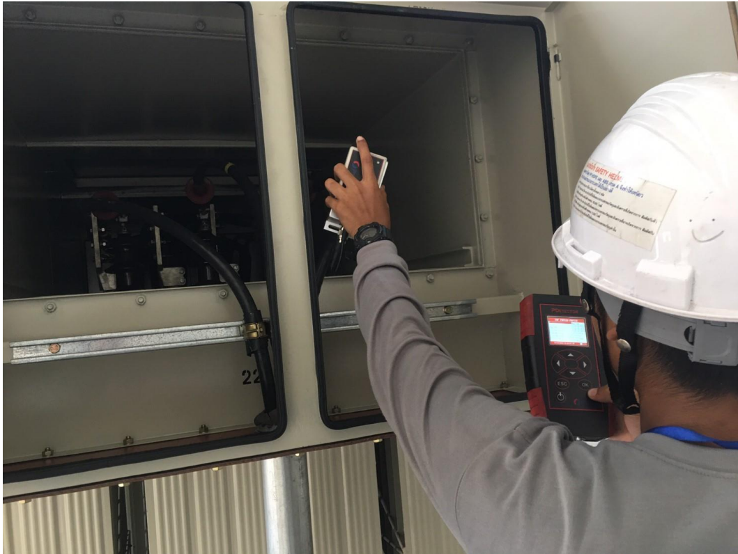
PHOTO 5 : PARTIAL DISCHARGE INSPECTION BY UHF MODE
