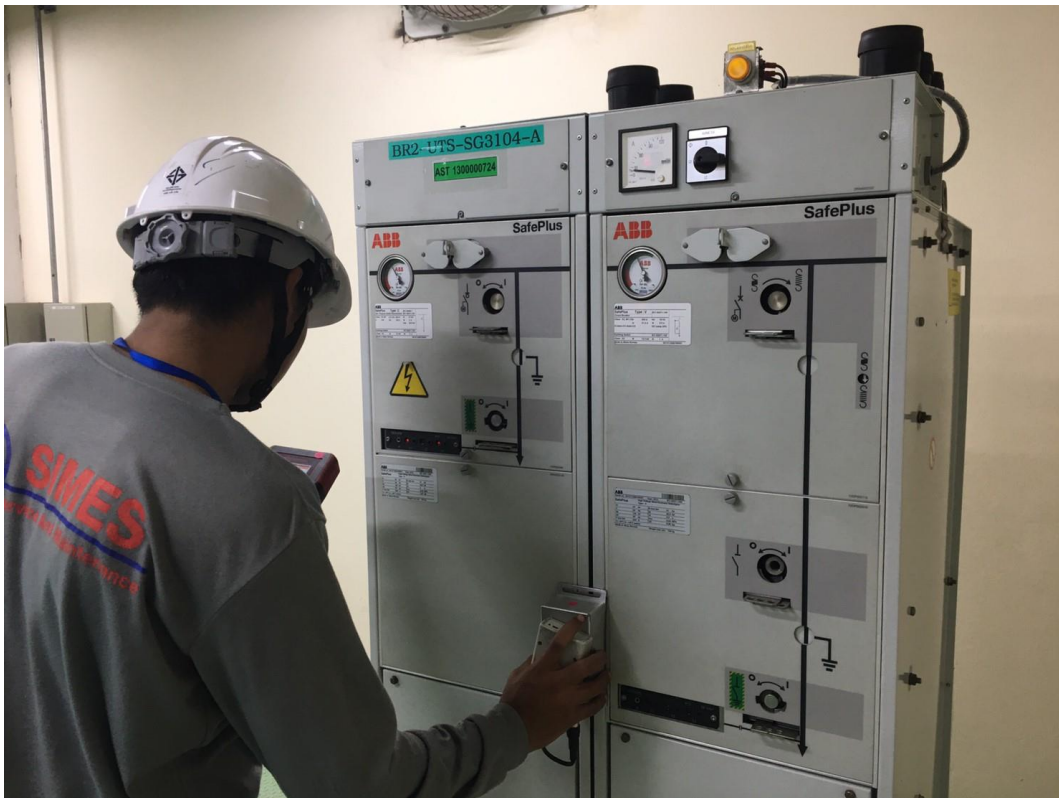
PHOTO 4 : PARTIAL DISCHARGE INSPECTION BY UHF MODE
