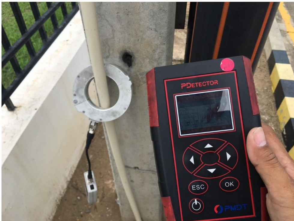
PARTIAL DISCHARGE DETECTED METHOD BY HFCT MODE
