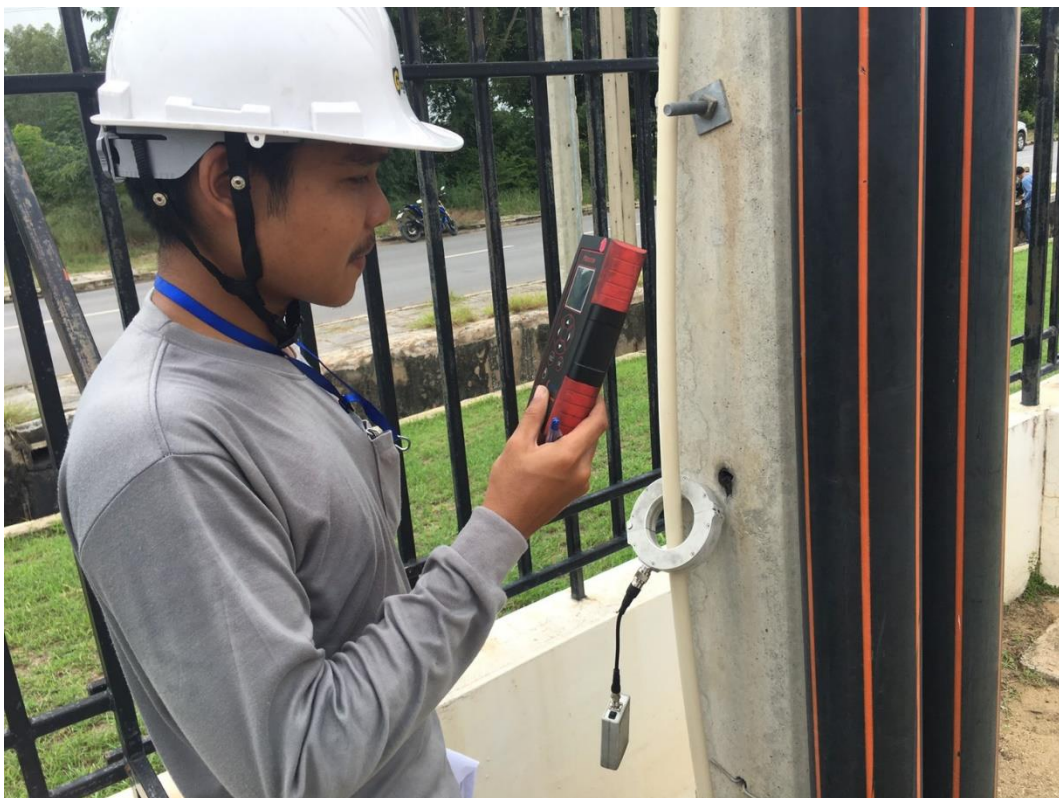
PHOTO 8 : PARTIAL DISCHARGE INSPECTION BY HFCT MODE
