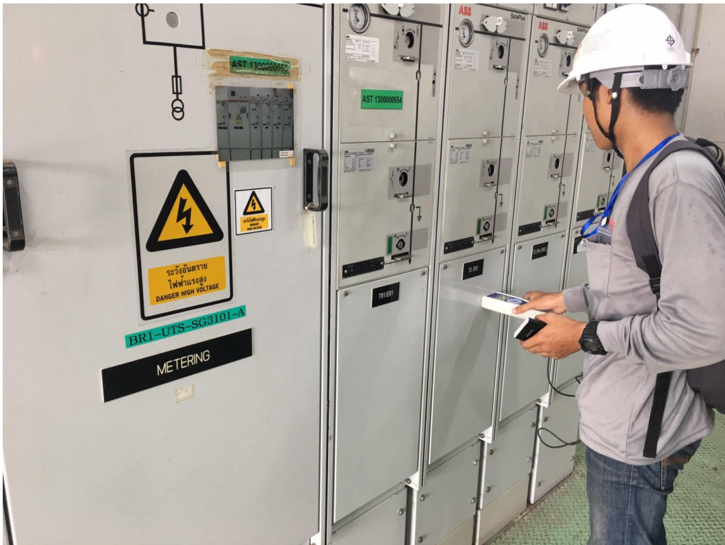
PHOTO 2 : PARTIAL DISCHARGE INSPECTION BY TEV MODE
